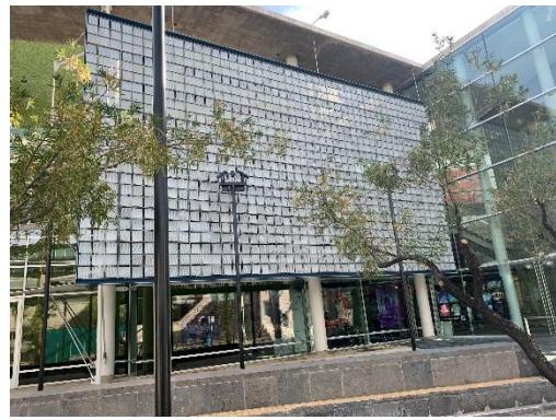
panel is made up of thousands of small blue aluminum panels that move with the wind, creating constantly shifting patterns that resemble ripples on water. The panels of the smaller screen are perforated with different sized holes that, when viewed from a distance, create a photographic image of sand dunes. Together these permanent installations comprise Fragmented Landscape by Ned Kahn.
