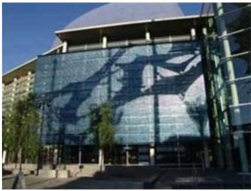
Two shade screens adorn the west-facing wall of the theater building, each consisting of thousands of small aluminum panels that are activated by wind. The larger
